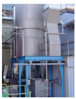
Venturi scrubbers offer more advantages in separating and recovering ultra-fine particulate and liquid mists than other gas-cleaning methods.
