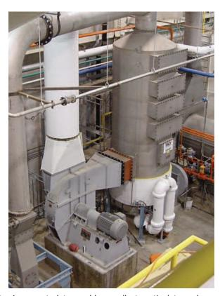
Impingement plate scrubbers collect particulate and absorb vapors and gases. High collection efficiencies (99+percent) can be achieved with low water consumption and minimum pressure drop.
